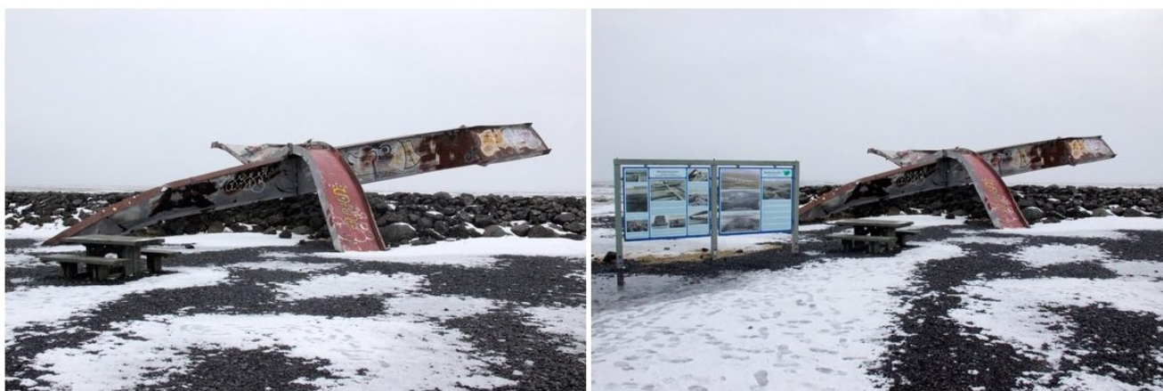
All that remains of the bridge is two girders entangled on the edge of the sandur plain. JACK YARWOOD [JACK YARWOOD/USED WITH PERMISSION ]
