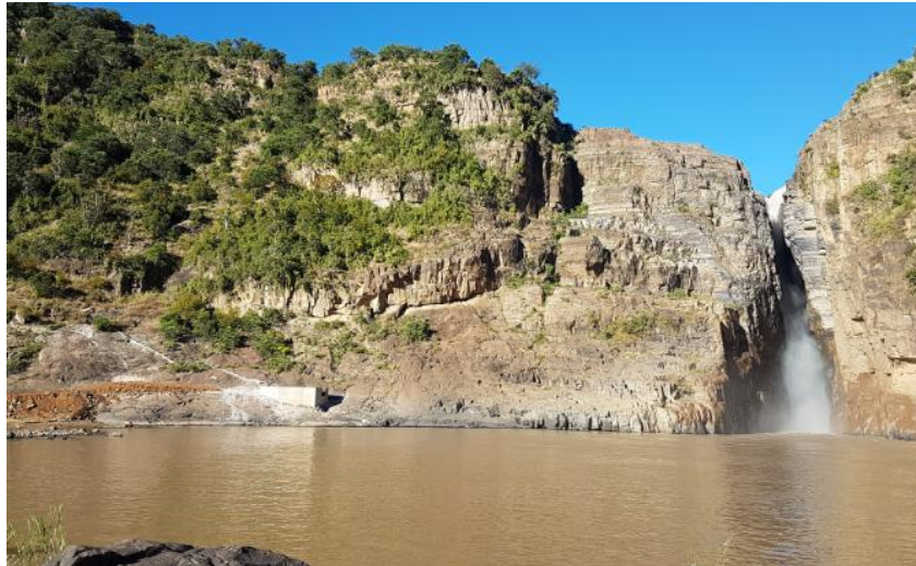
The Thina waterfall. The concrete structure at the left is part of a hydroelectric micro-power station, under construction at the time of the photo.
