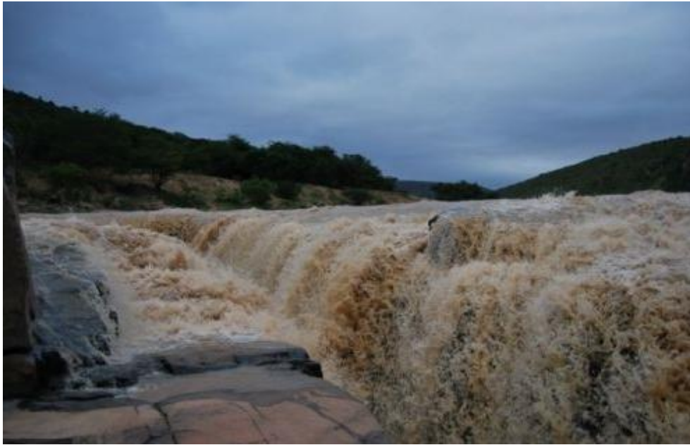
At the top of the waterfall, the water drops into the trench, making the rather unusual sight of a pair of waterfalls facing each other, about 2 metres apart.
