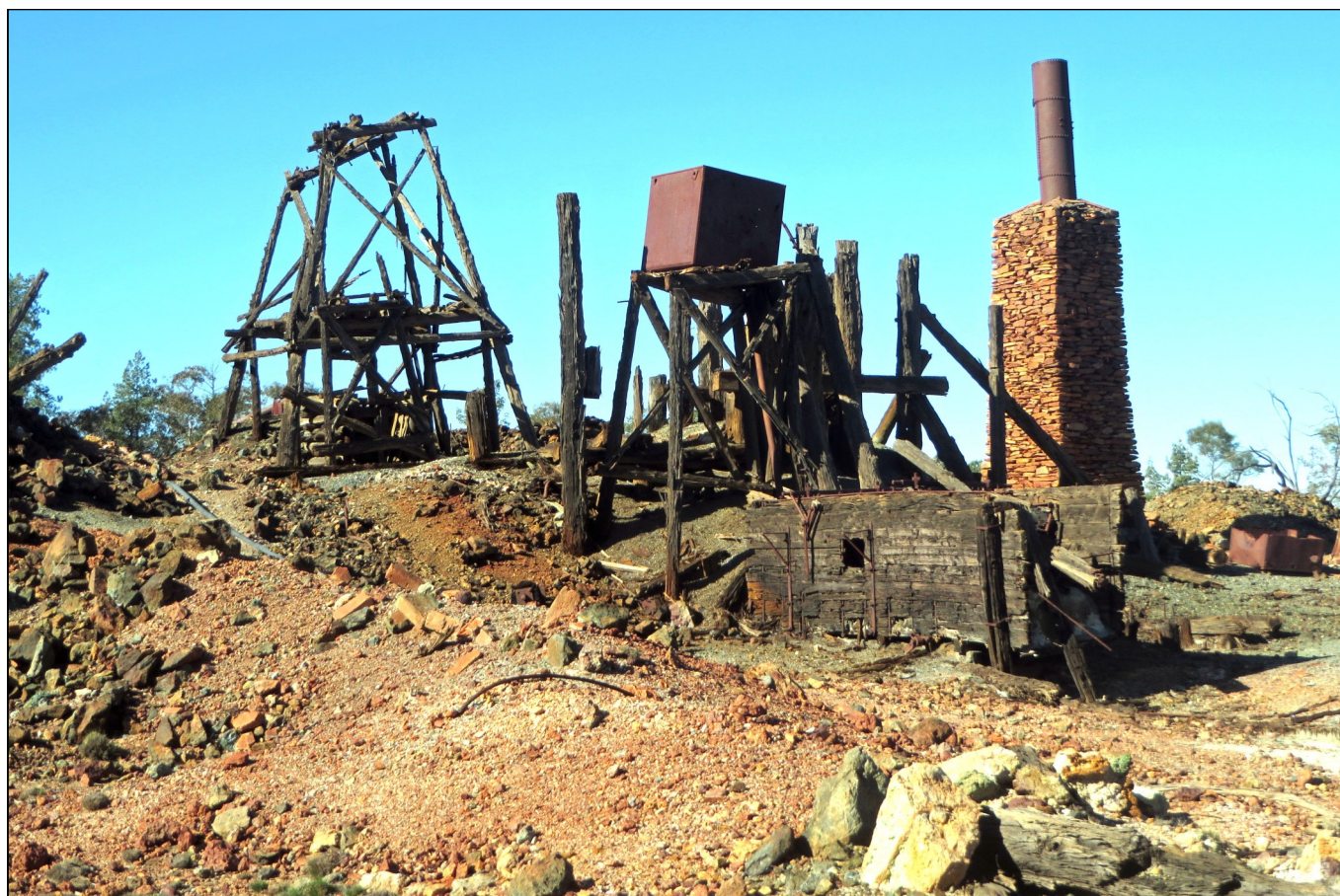
49. Left to right: Headframe of Hodges main shaft, square water tank that fed the rectangular wooden Hancock jig situated below the drystone chimney and water tank.
