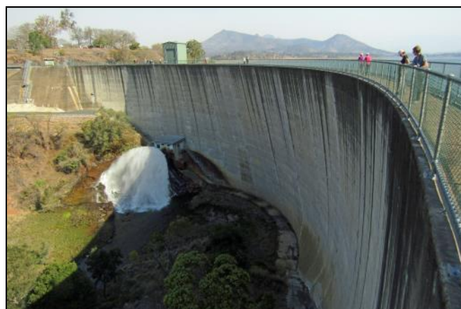
54. Double concrete curvature wall of Moogerah Dam.
