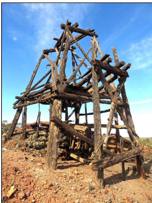
48. Cyprus headframe of the Hodges Main shaft at the Great Central mine.
