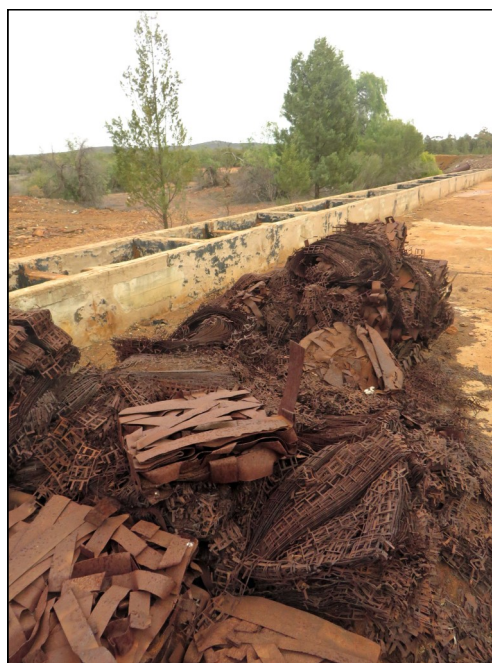
25. Row of concrete tanks used in the mid 1950's to extract copper from mine water by the cementation process. Note the piles of scrap iron used for precipitation.
