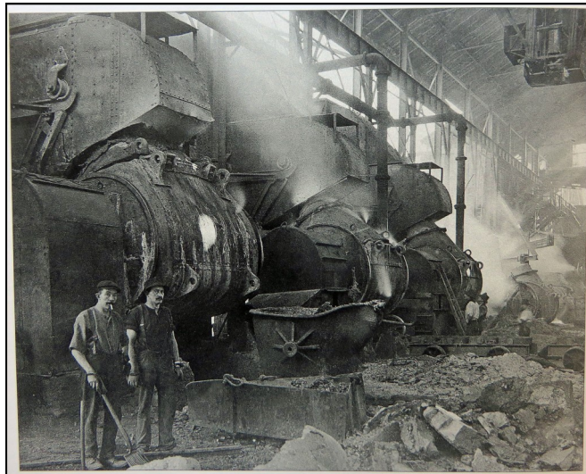
4. Two of the Bessemer converters in operation at the Great Cobar Smelter.
