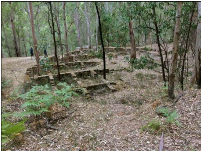
35. Circular brick foundations for one of the many large steel storage tanks.
