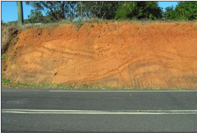
25. Road cutting of Landsborough Sandstone. Note the folding and faulting in the exposure.
