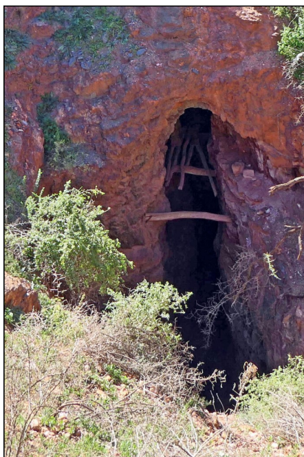
6. Historic workings near the Chesney No. 2 shaft. Note the remnants of the timber working platform.
