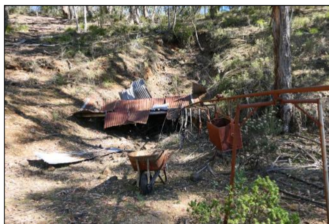
7. Katos Adit today showing detail of monorail system to carry excavated rock out of adit. Photo Ron Evans.
