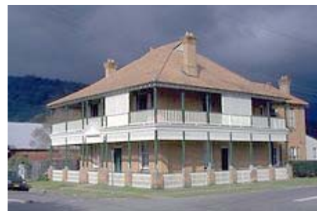
The former CBC Bank designed by G.A. Mansfield and built 1897-1902
