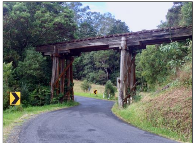
25. Abandoned historical wooden rail bridge on Coramba Road near Megal.
