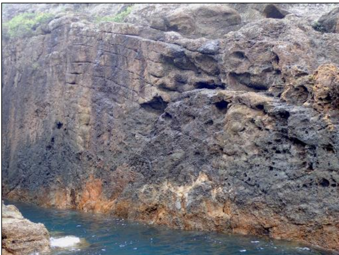
11. Conglomerate wall beside the eroded dyke.
