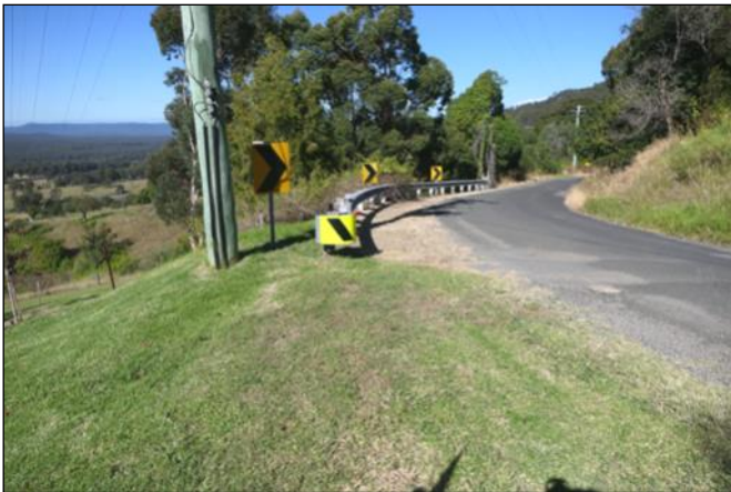
10. The section of road running down the slope follows the Mount View/Paxton fault. Because it's a normal fault, the land to the left has dropped down with respect to the land on the right.
