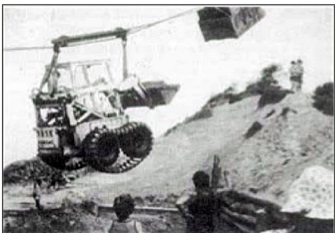
4. Bobcat and skip used by Mr Frisby to collect pebbles from the sea cave at Snapper Point.
