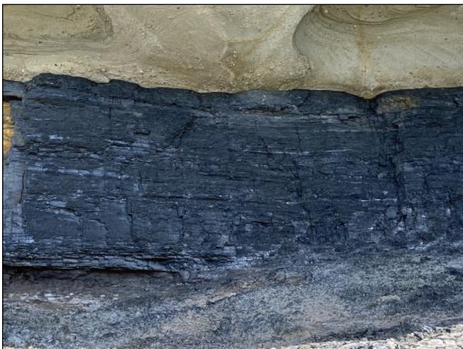
18. Erosion on the surface of the Vales Point coal is obvious when looked at closely.
