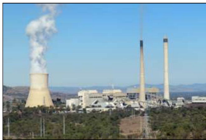
57. Callide Power Station.
