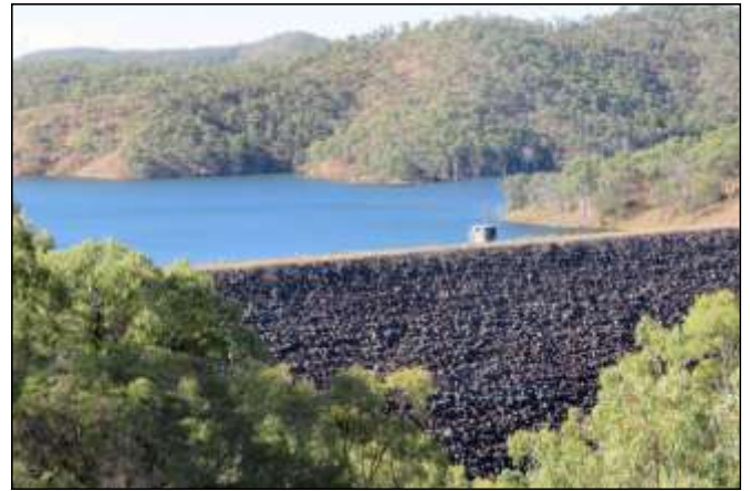
39. Cania Dam wall.
